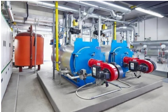
Boiler Conversion & Modification
