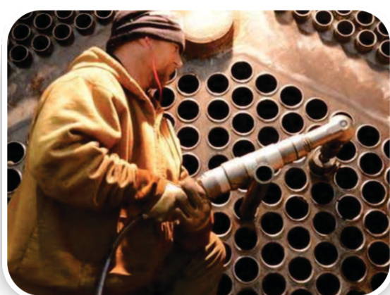
BOILER TUBE REPLACEMENT
